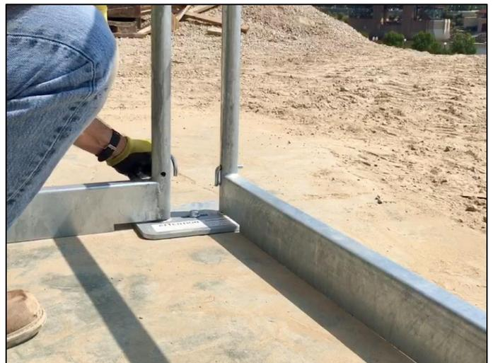
**Step 3:** Set guardrail section on baseplate.
