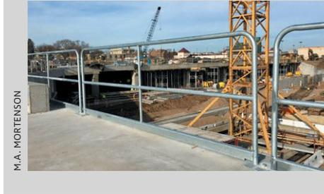
The guardrail system has been deployed on three M.A. Mortenson-partnership projects and has eliminated 80,000 linear ft of wood guardrail and reduced 60% of installation and maintenance labor. No injuries have been reported during installation and handling.
